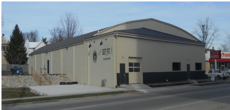
Renovated former Fisher Lumber building – Get Fit LLC
